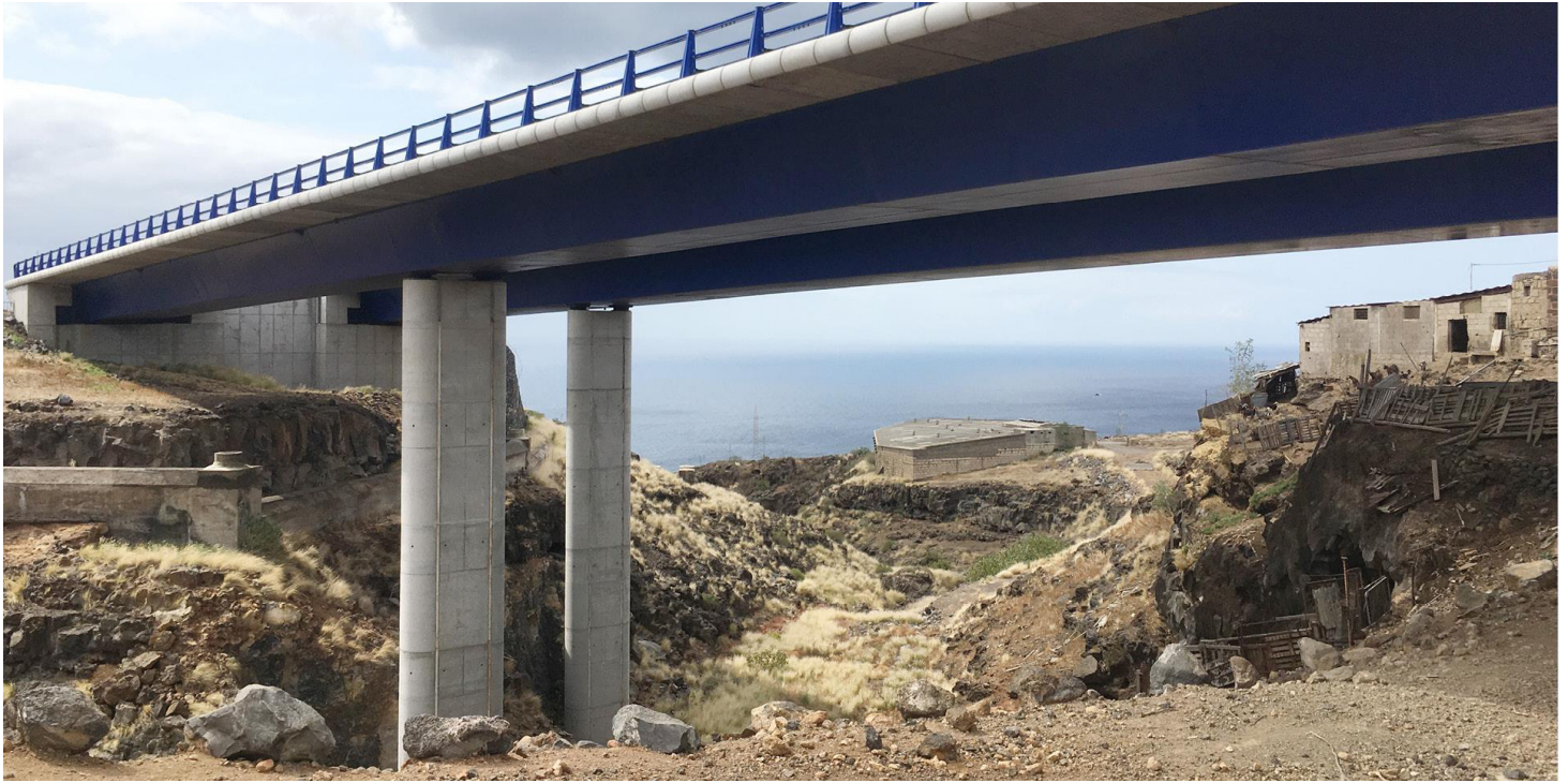
Composite double deck viaducts with 92m total length each / Main span: 63.5
